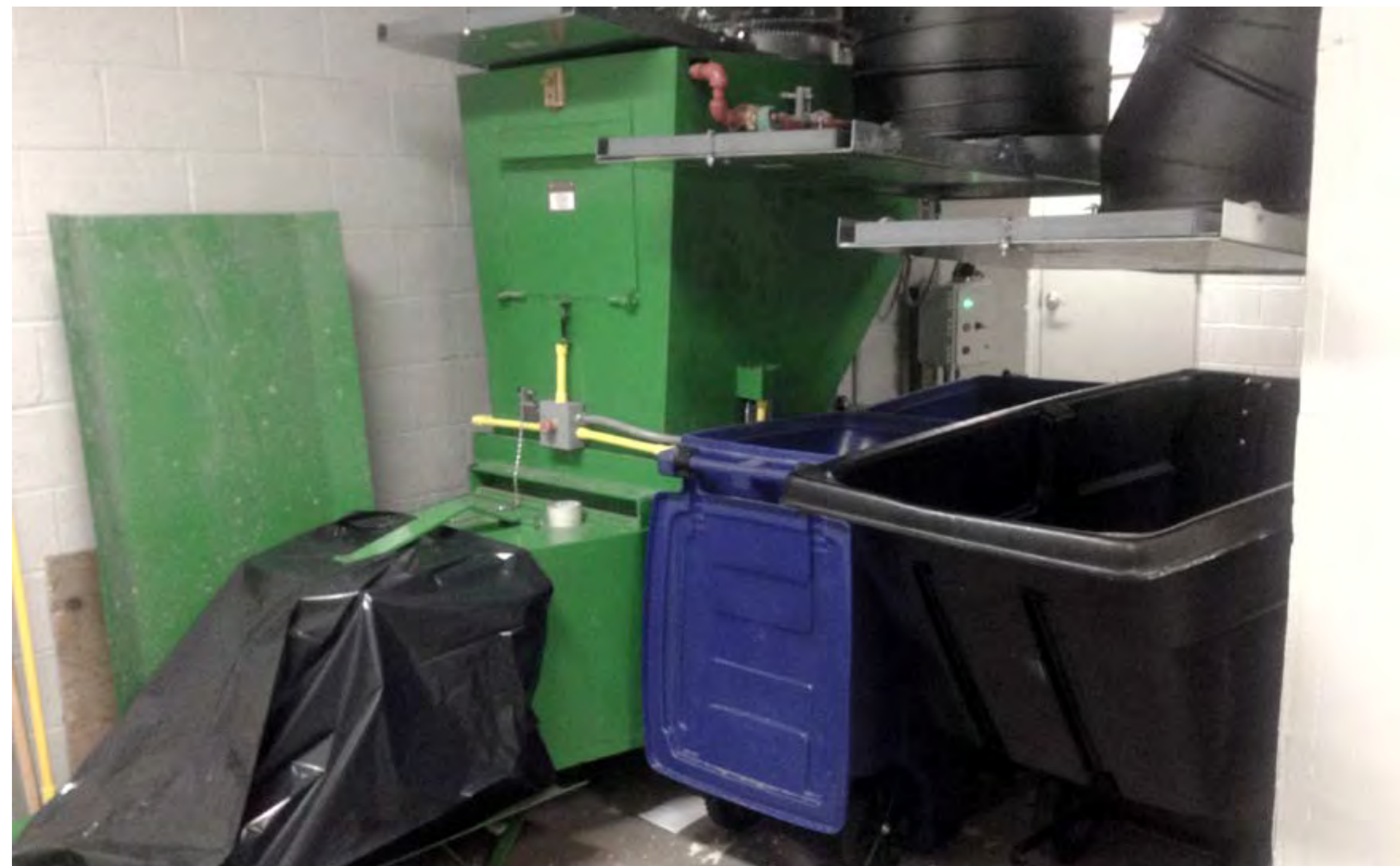
Top to bottom: Multiple chutes to wheeled bins; Multiple chutes to 2 cu yd containers
