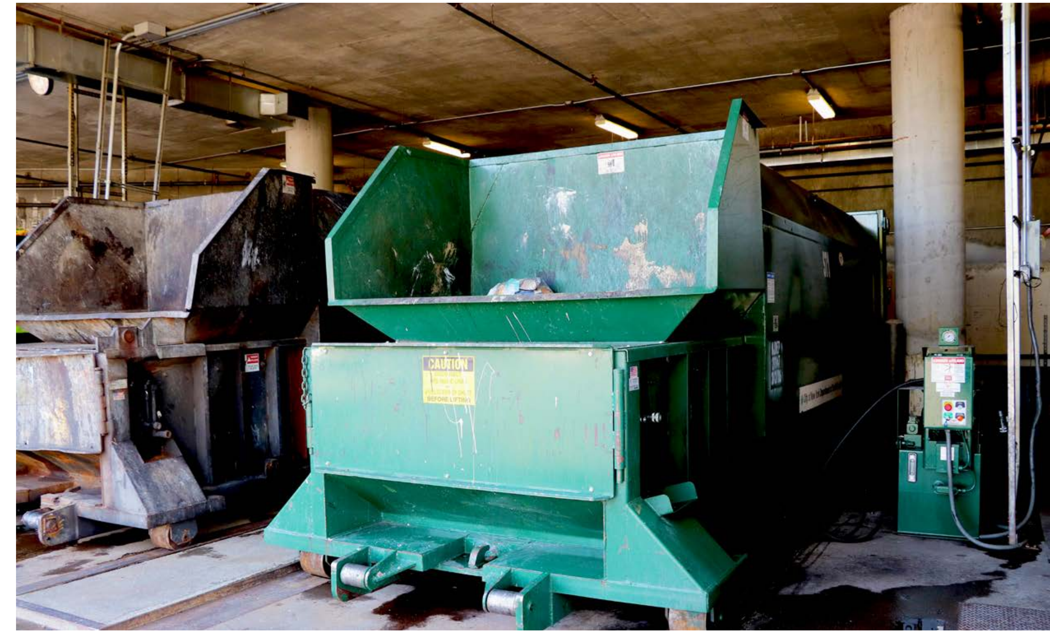
Stationary compactor with hopper feed (collected by DSNY)
