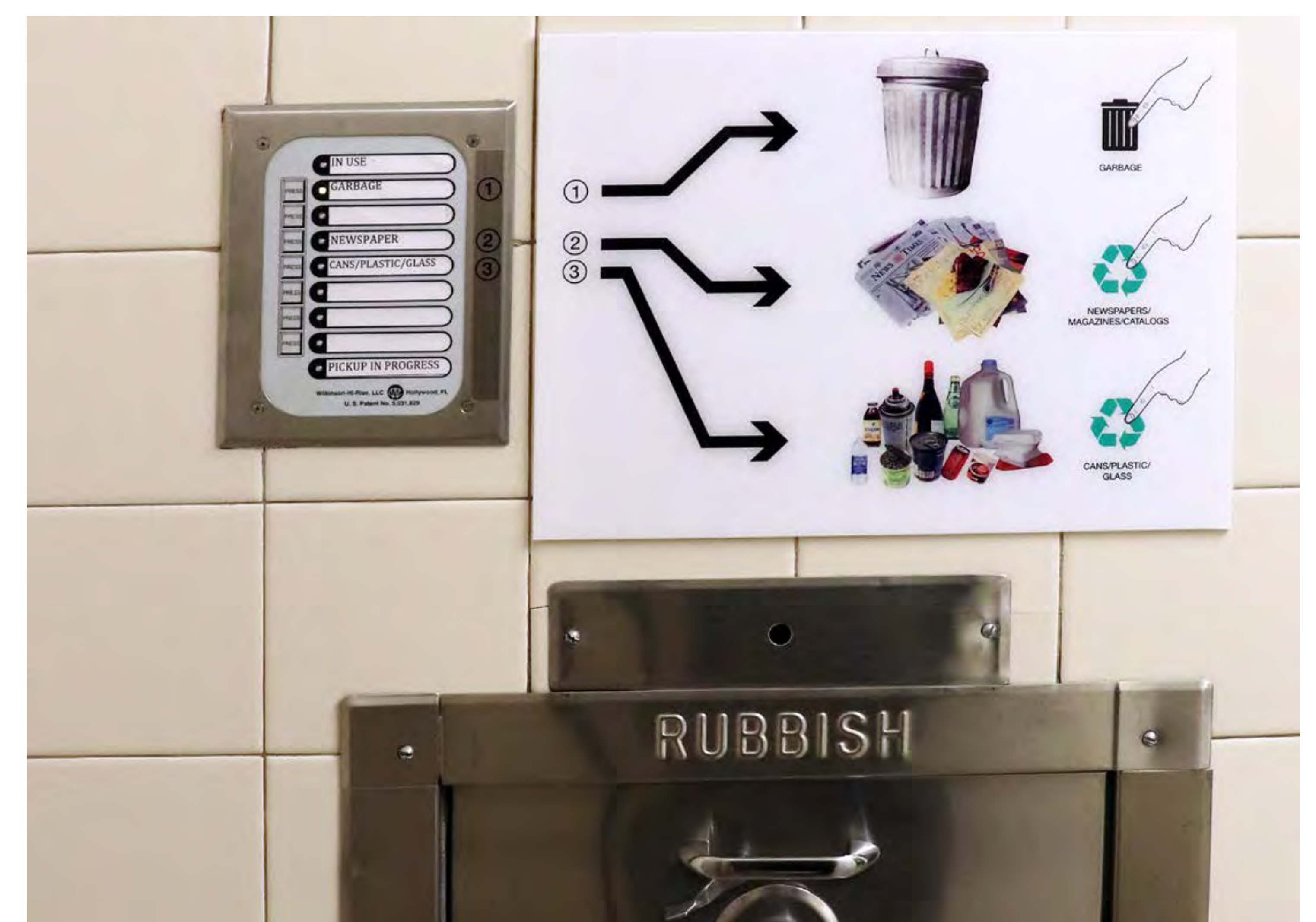
Control panel for residents to select waste streams for bisorter and turntable; Chute to bi-sorter with compactor and turntable
