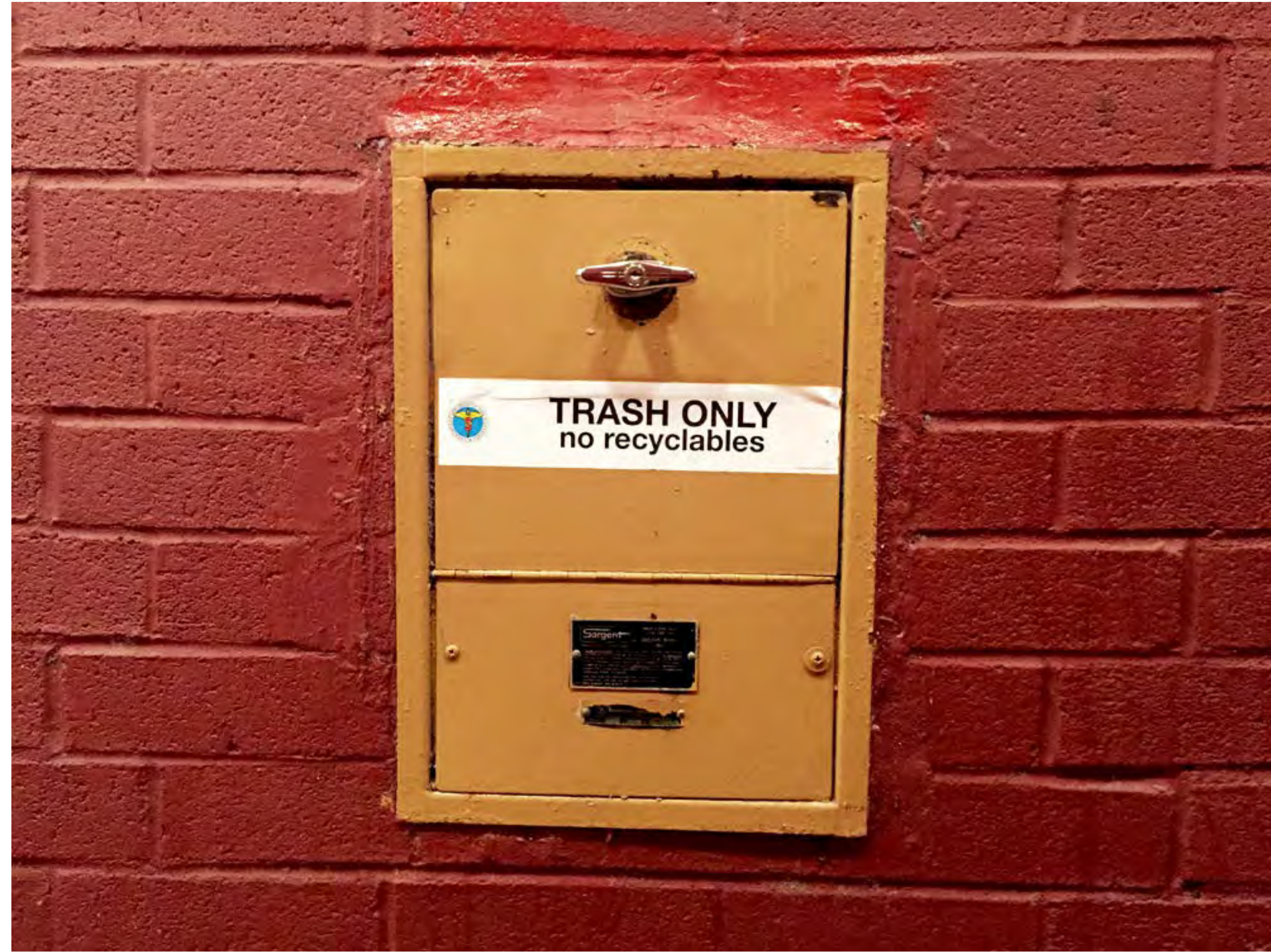
Chute door in residential corridors and central recycling station
