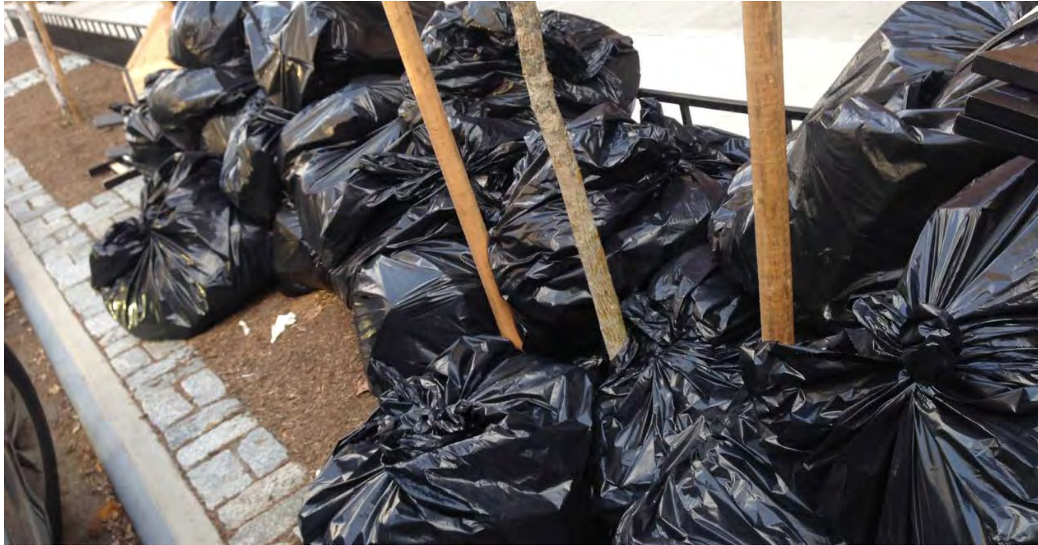
Elongated tree pit for stormwater infiltration with no space for waste setout
