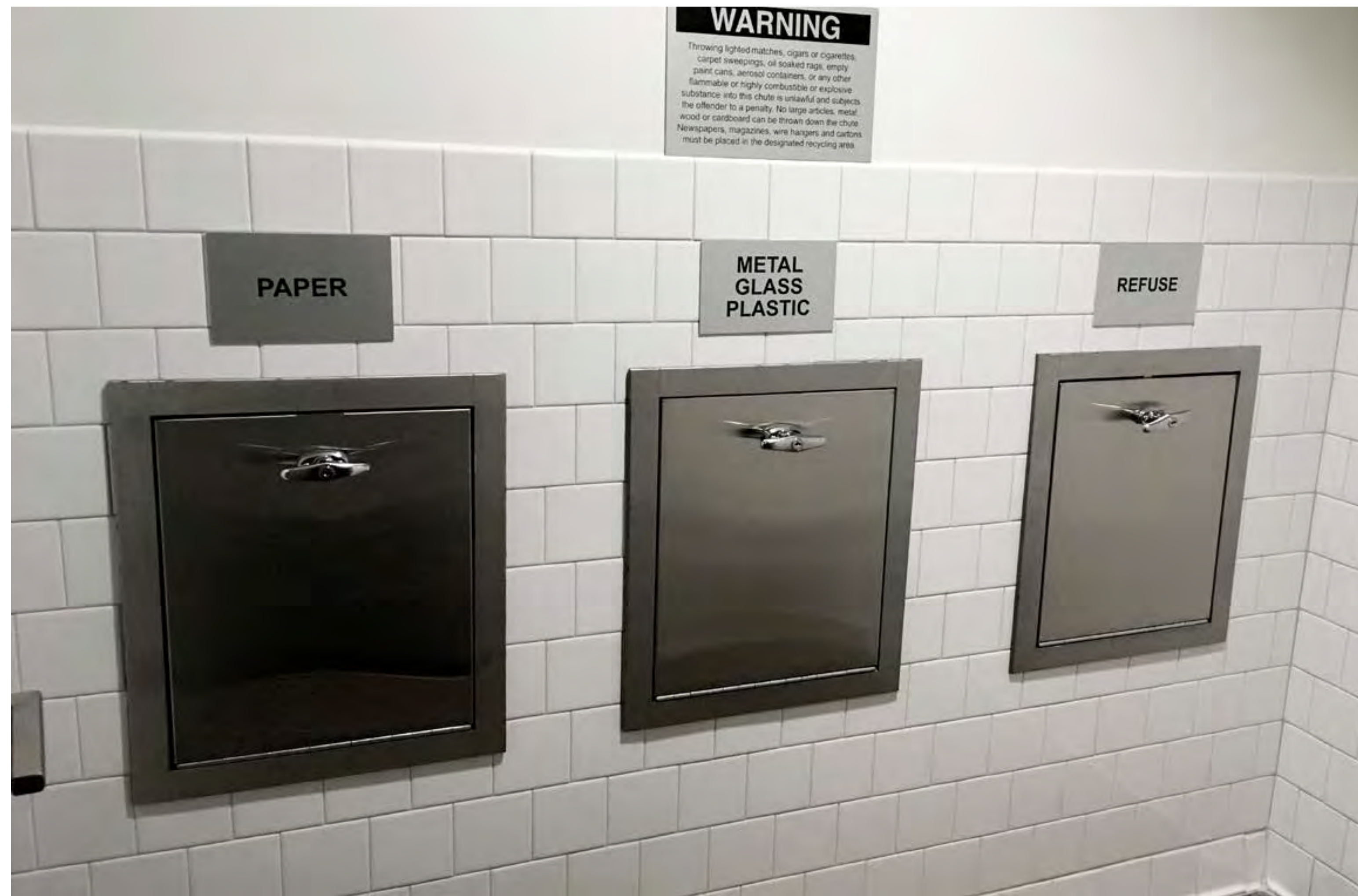
Three separate chute doors for trash, MGP and paper
