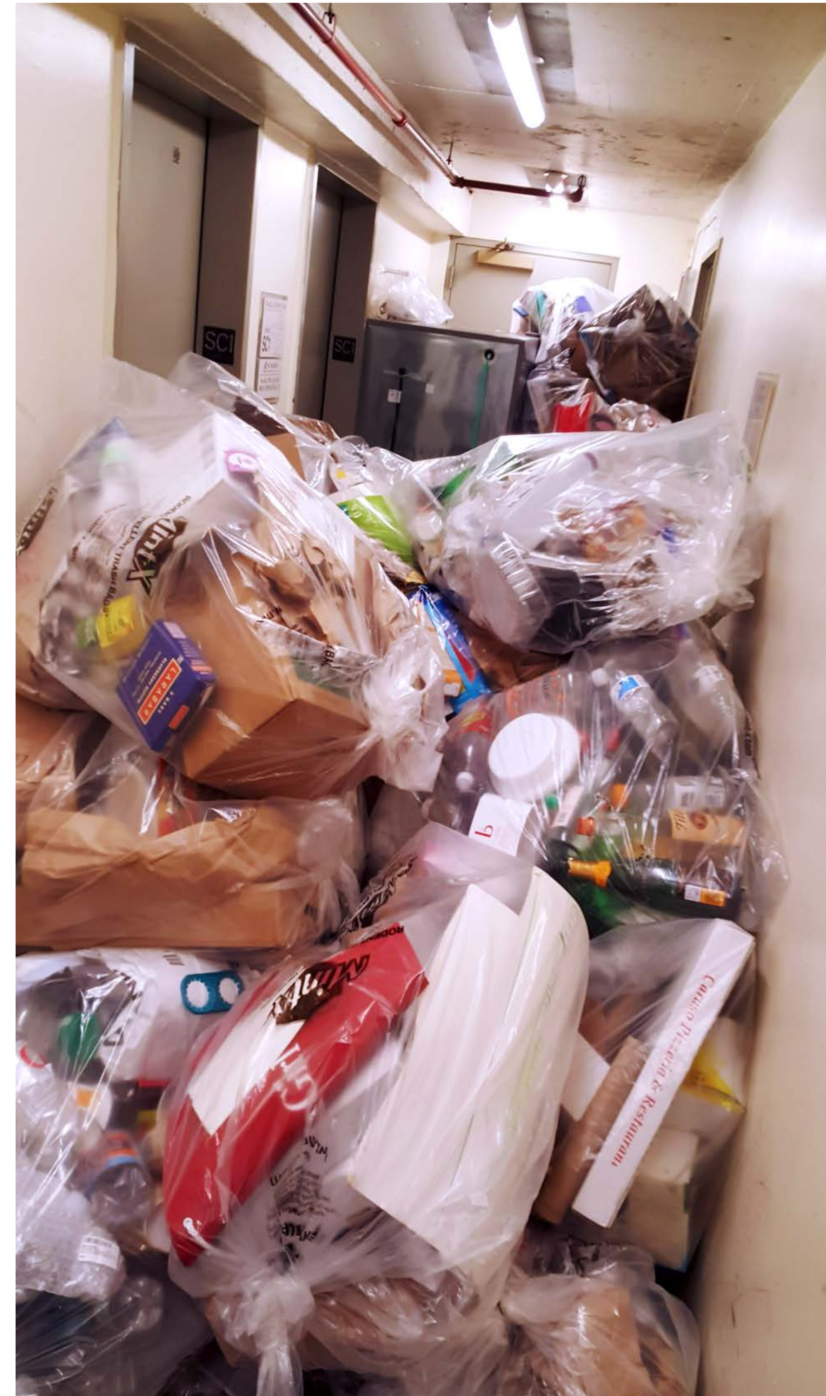
Recyclables blocking egress corridor
