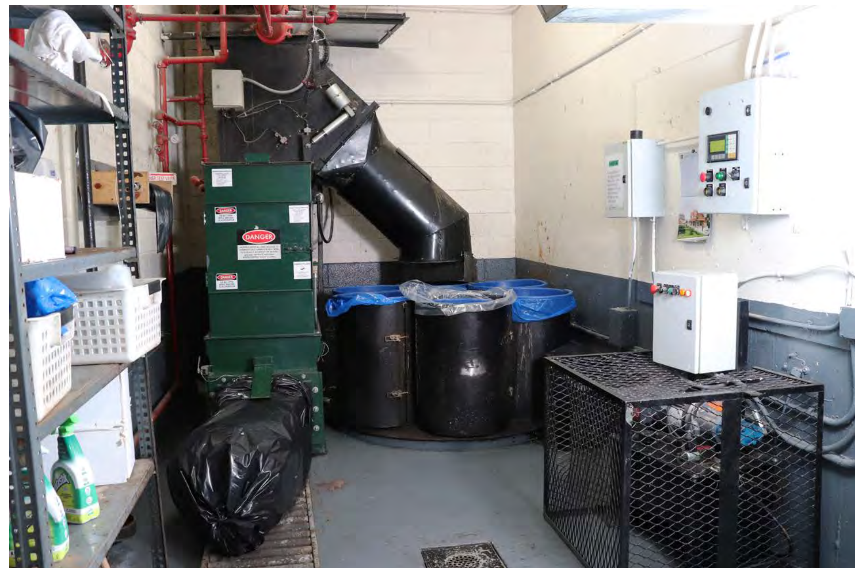
Control panel for residents to select waste streams for bisorter and turntable; Chute to bi-sorter with compactor and turntable
