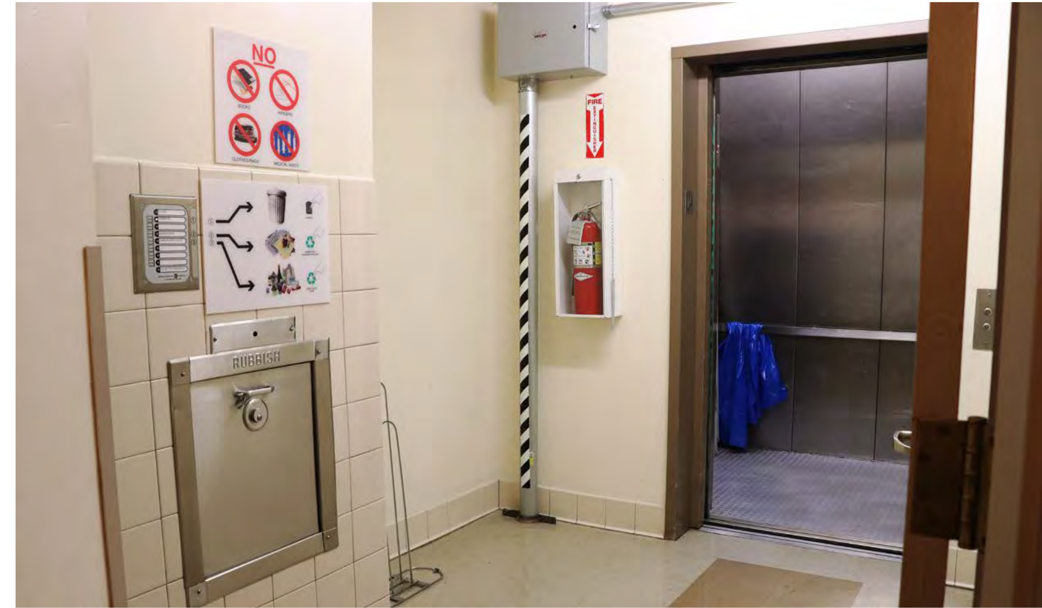
Above: Waste room with chute door, sorter control panel and service elevator access
