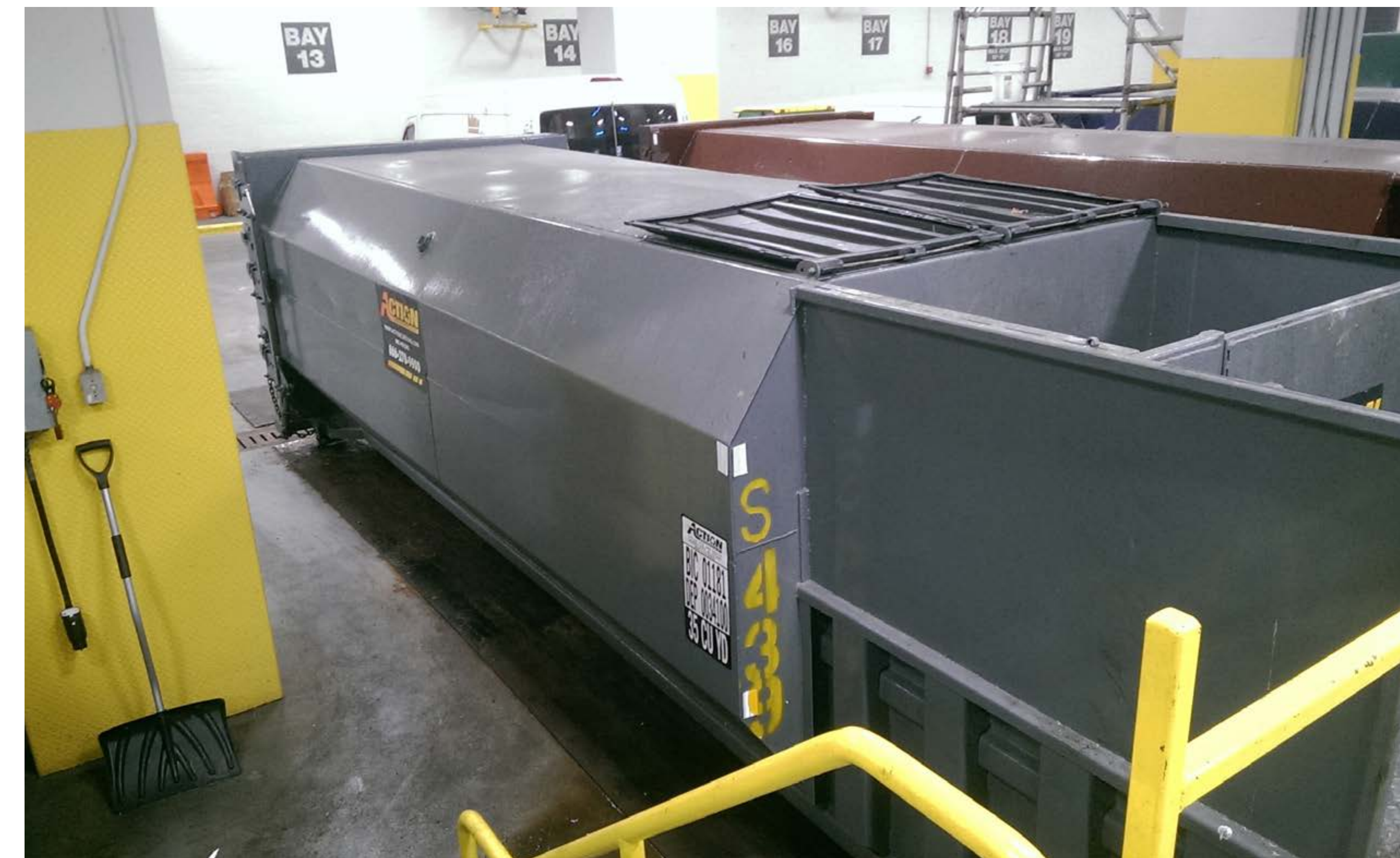
Self-contained compactor in loading dock
