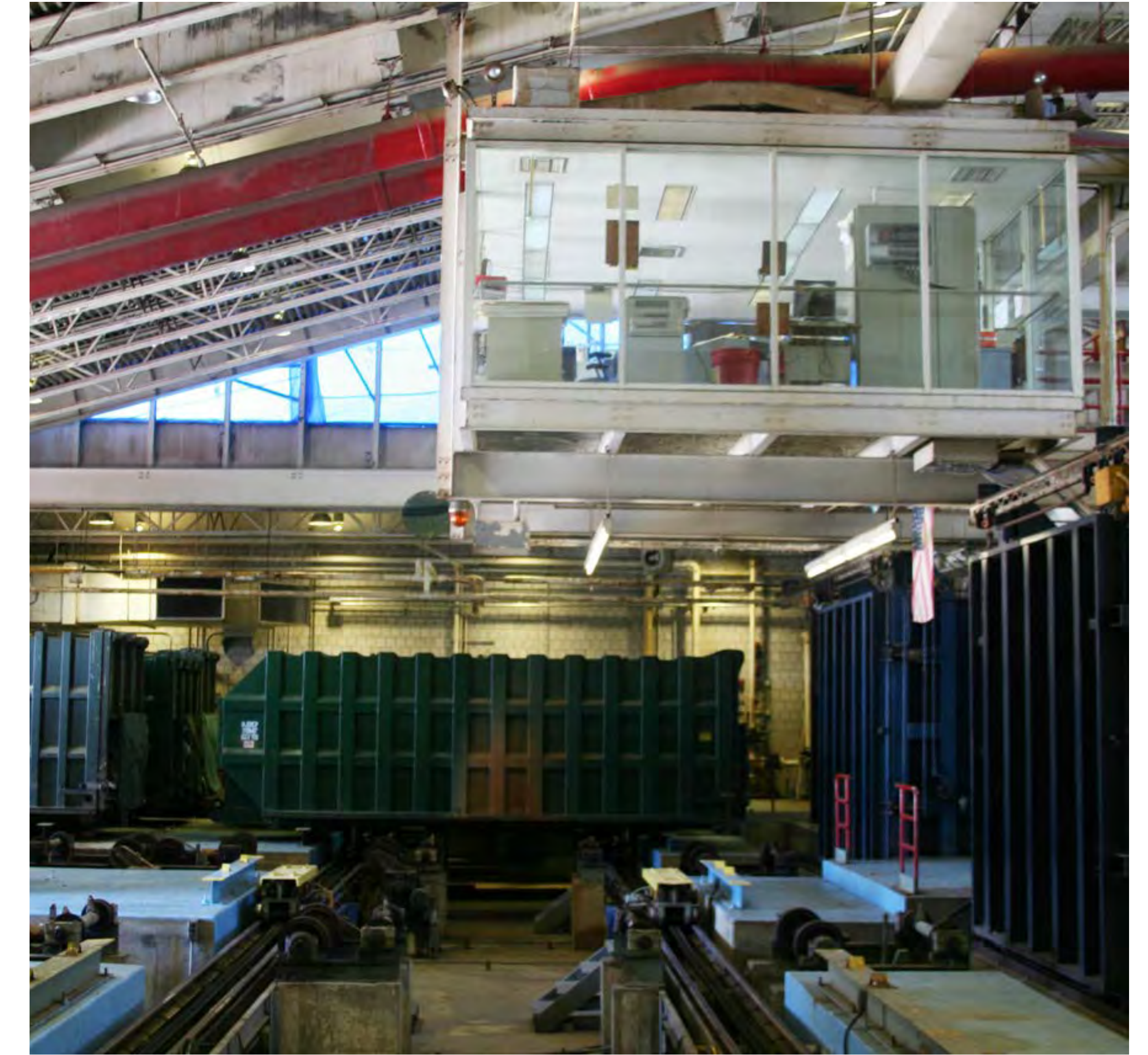
A valve in the building cellar at the base of a gravity chute connects to the pneumatic tube below; View inside the terminal (pneumatic tubes are painted red) including container moving equipment for 30 cu yd containers
