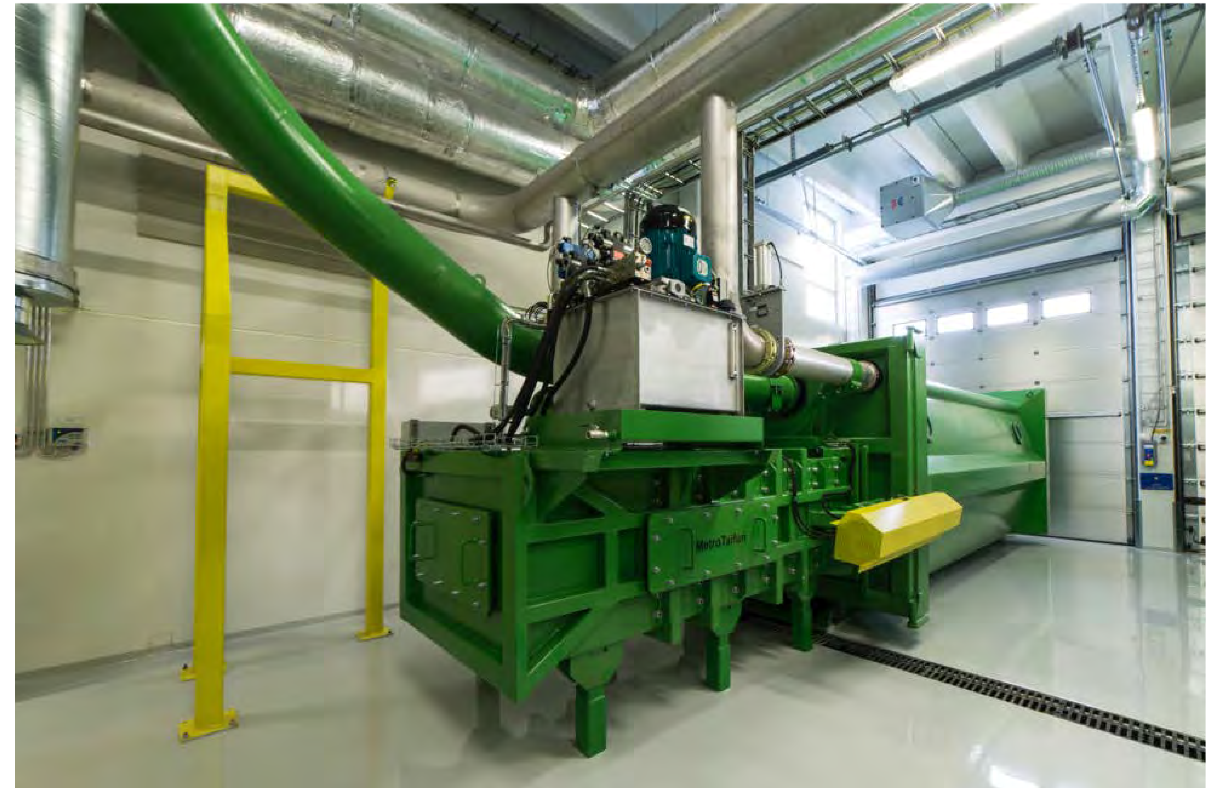
Above: Compactor container fed by pneumatic tube
