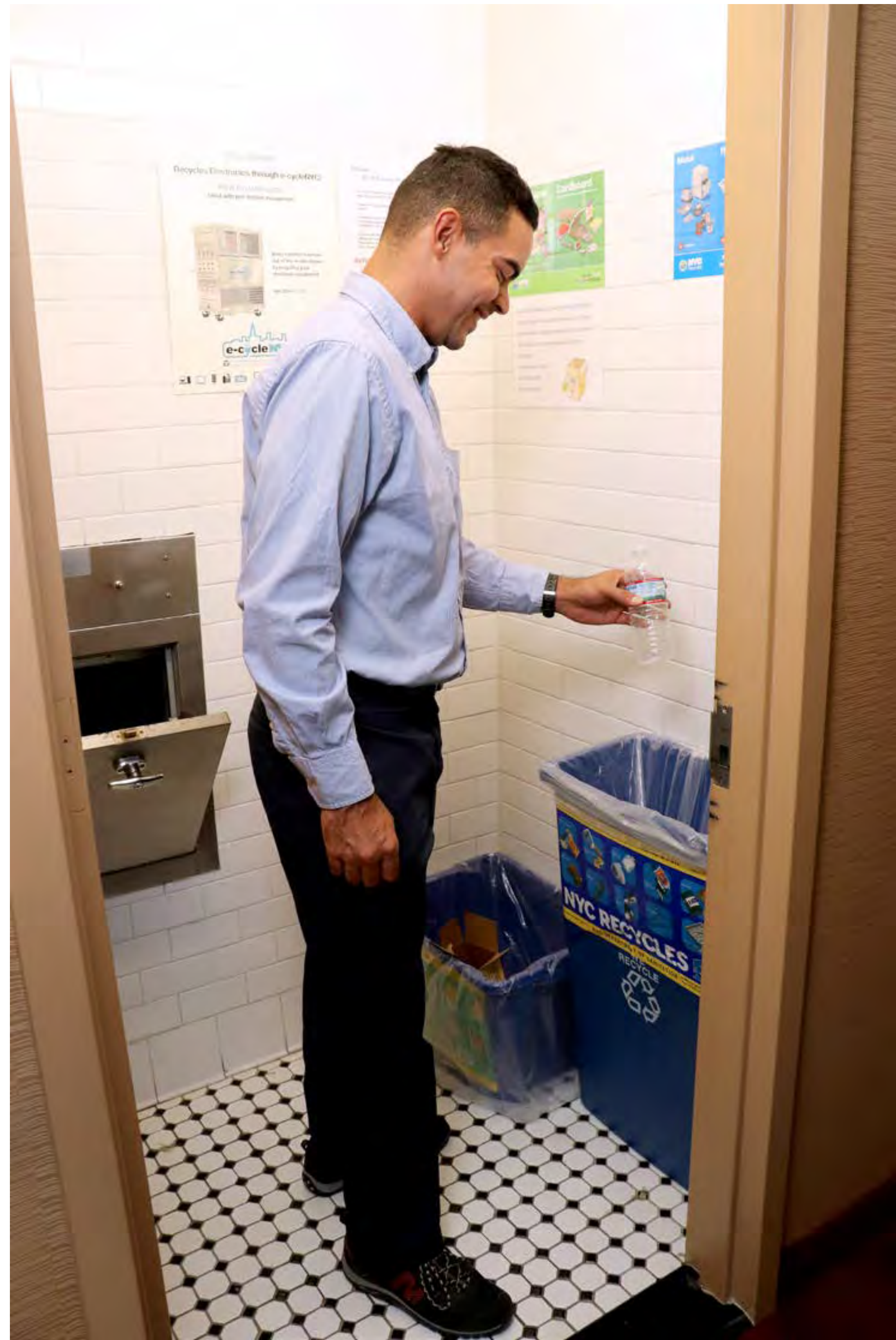
Waste rooms are typically small and unventilated, with chute access and recycling bins; Trash chute connected to compactors with “sausage” bags.
