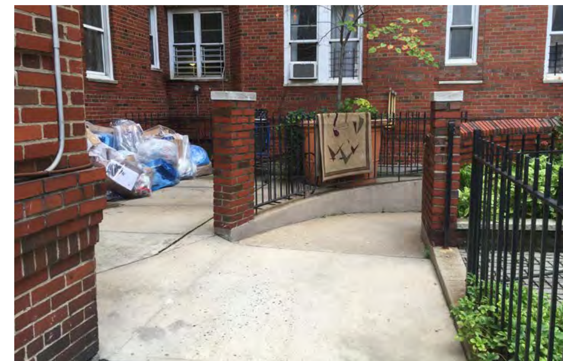
A semicircular ramp is designed into the exterior court, allowing waste to be wheeled from the basement to the sidewalk
