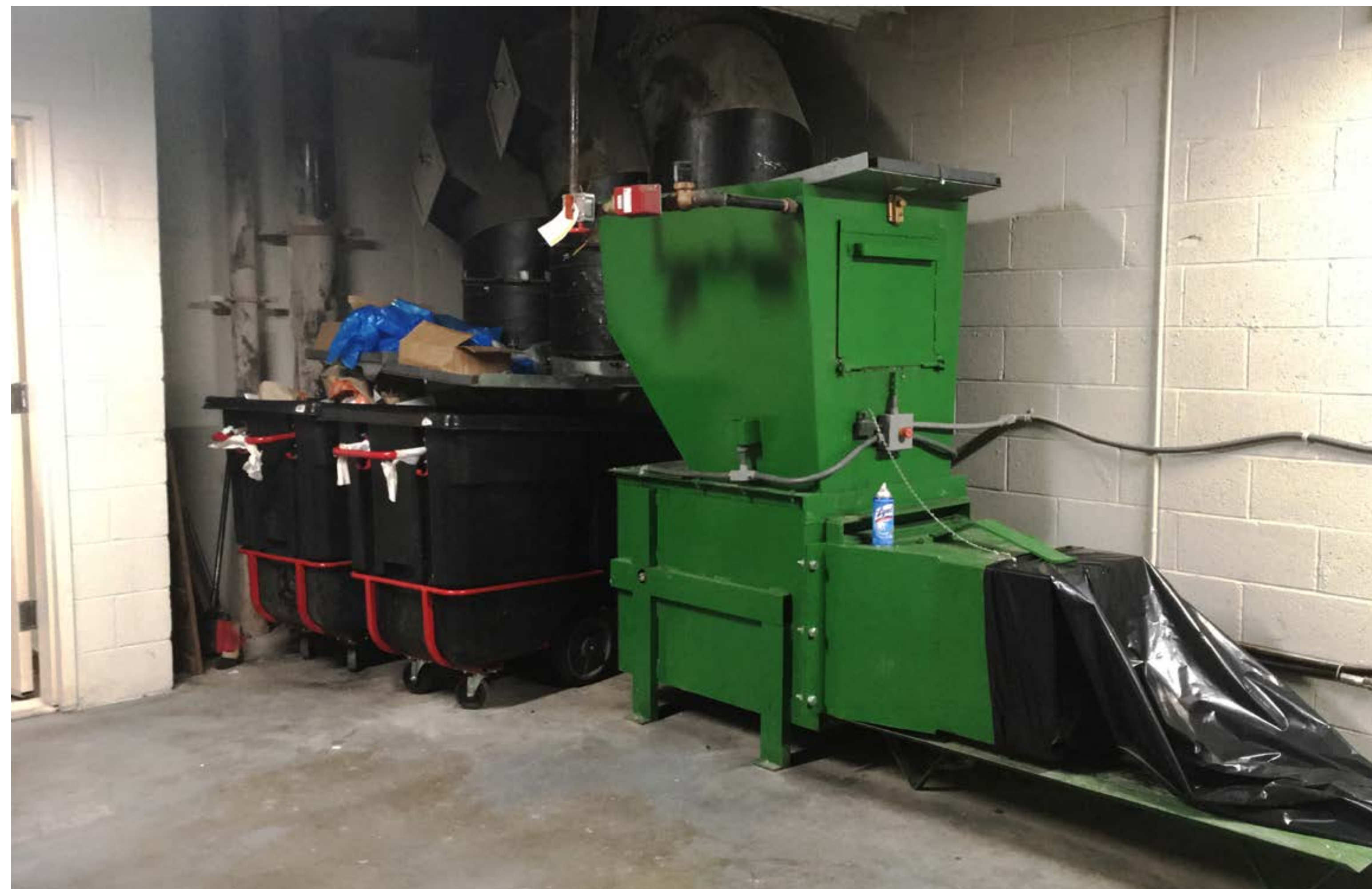
Trash chute empties into a compactor; MGP and paper chutes empty into tilt trucks
