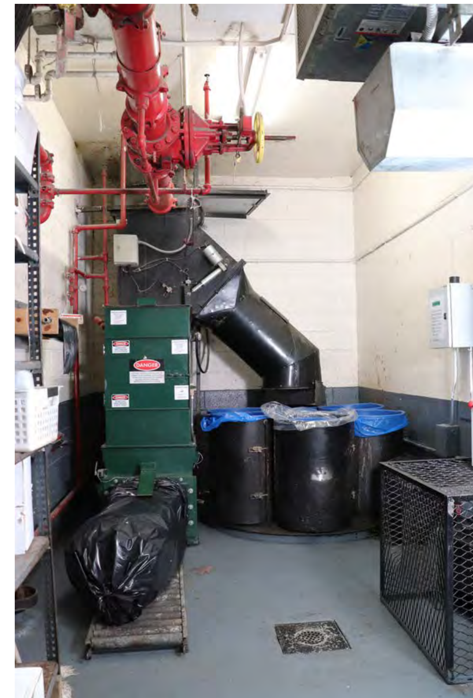
Above: Waste room with chute door, sorter control panel and service elevator access
