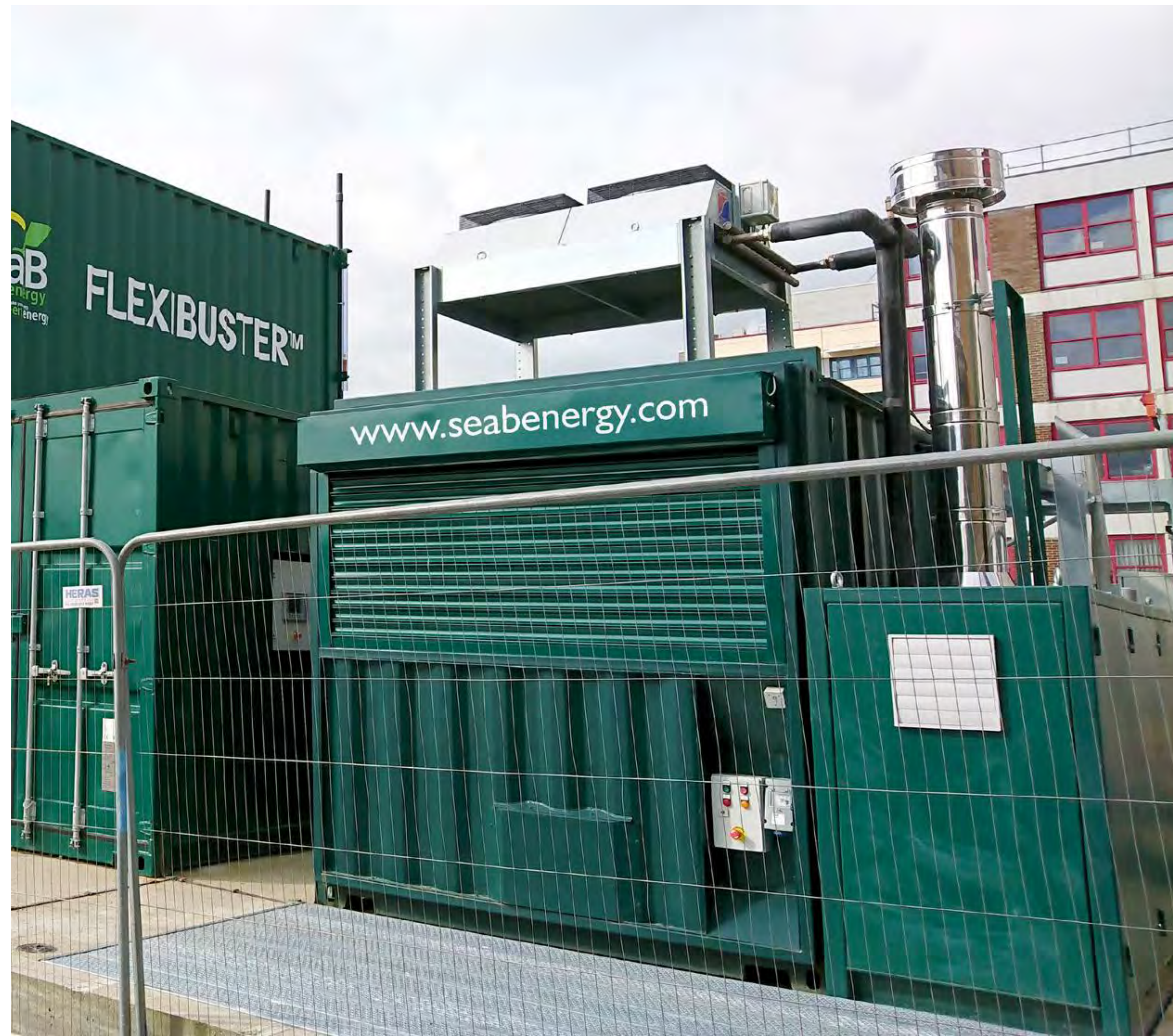
Anaerobic digester (SEaB Energy pictured)
