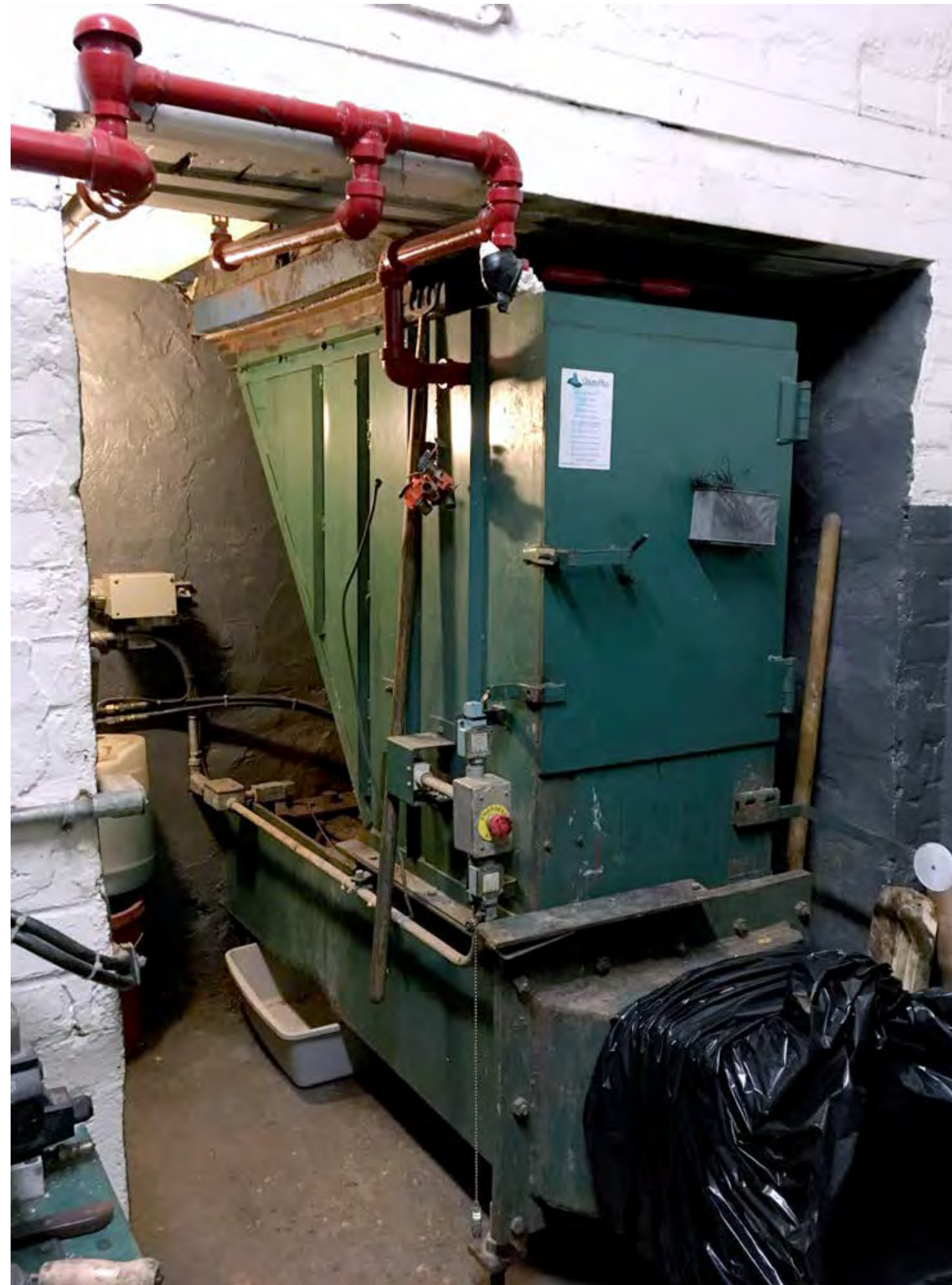
Converted chute with a compactor replacing the former incinerator.
