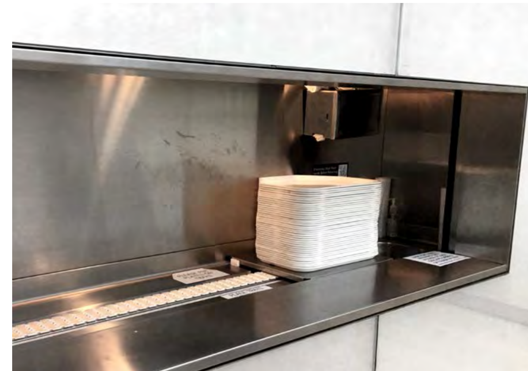
This dish carousel transports dishes, via a conveyer belt, from the second floor restaurant down to a dishwasher in the cellar.
