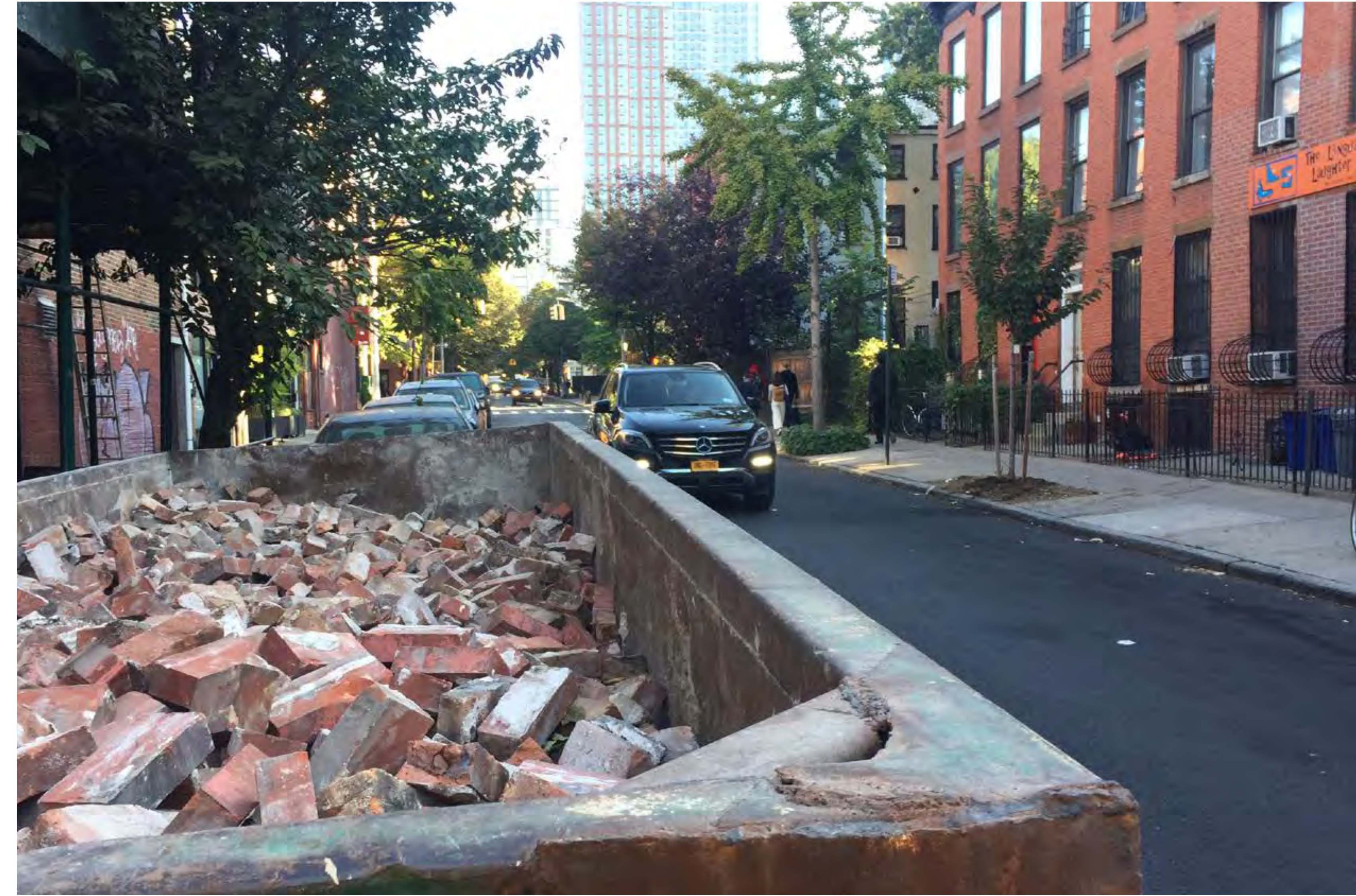
Salvaged bricks are separated for reuse
