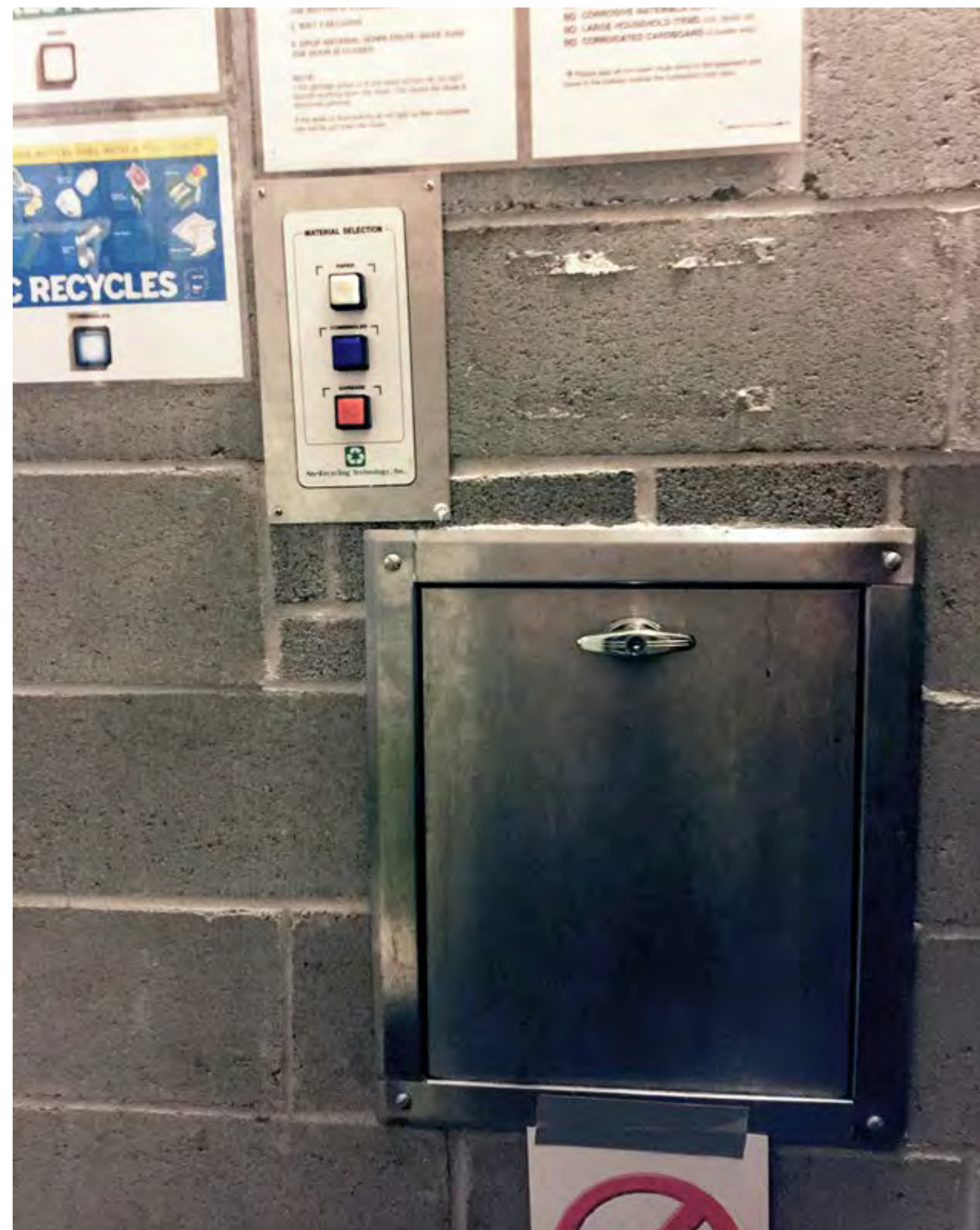
Simple 3 button control panel for trisorter; Chute to tri-sorter
