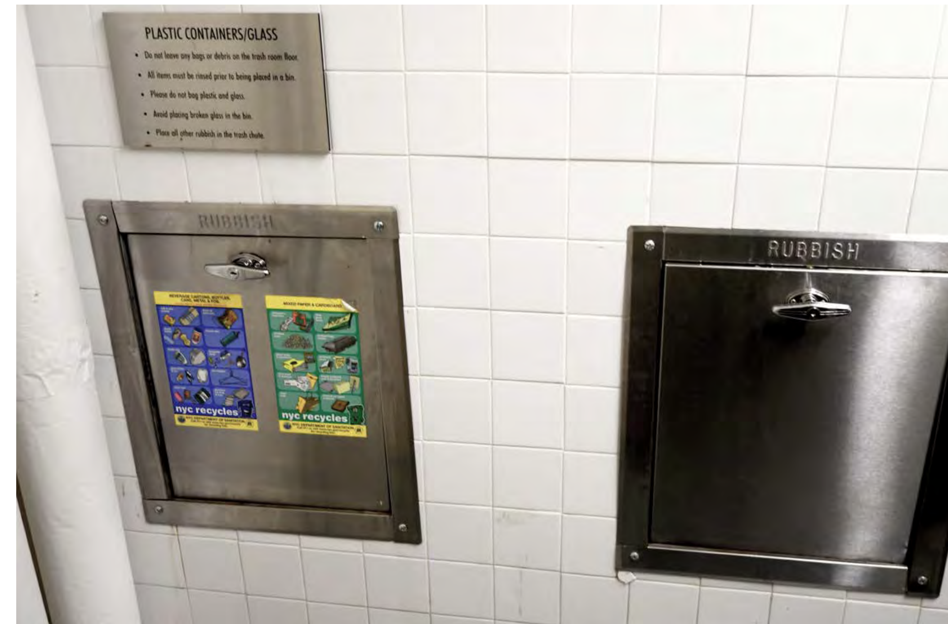
Two chute doors for trash and single stream recycling (private hauler collection)
