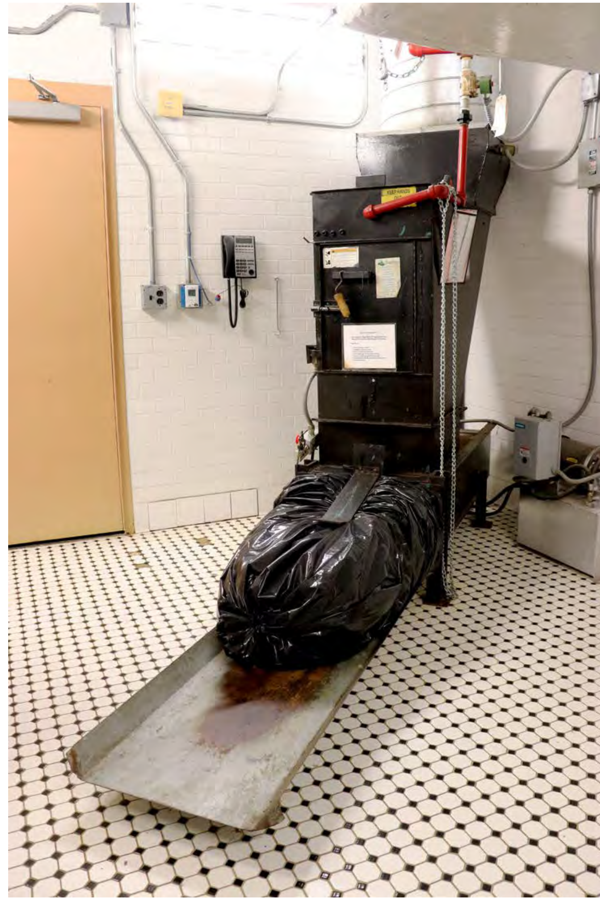
Waste rooms are typically small and unventilated, with chute access and recycling bins; Trash chute connected to compactors with “sausage” bags.
