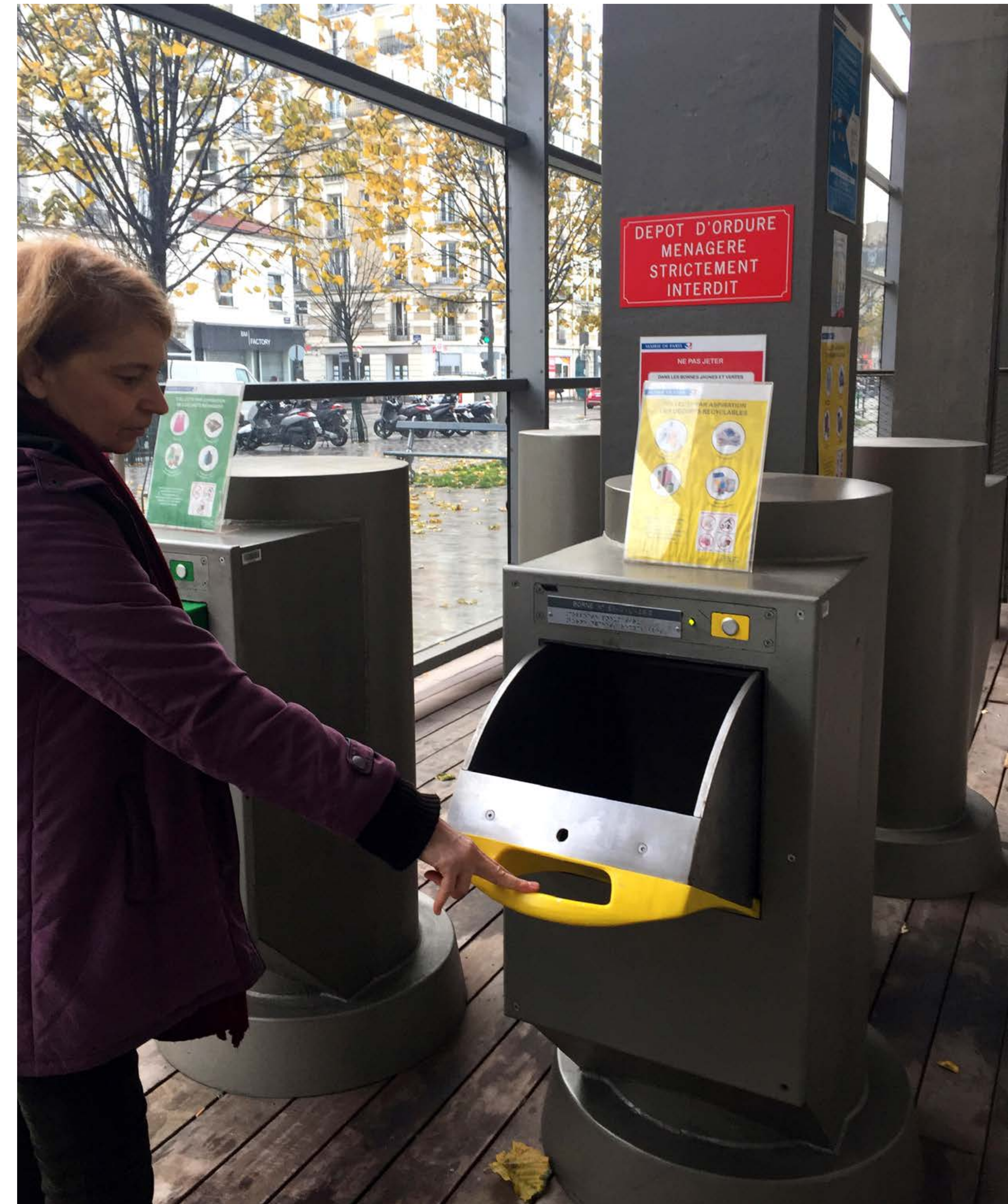
153 bis rue Cardinet pneumatic inlets for residents and daycare
