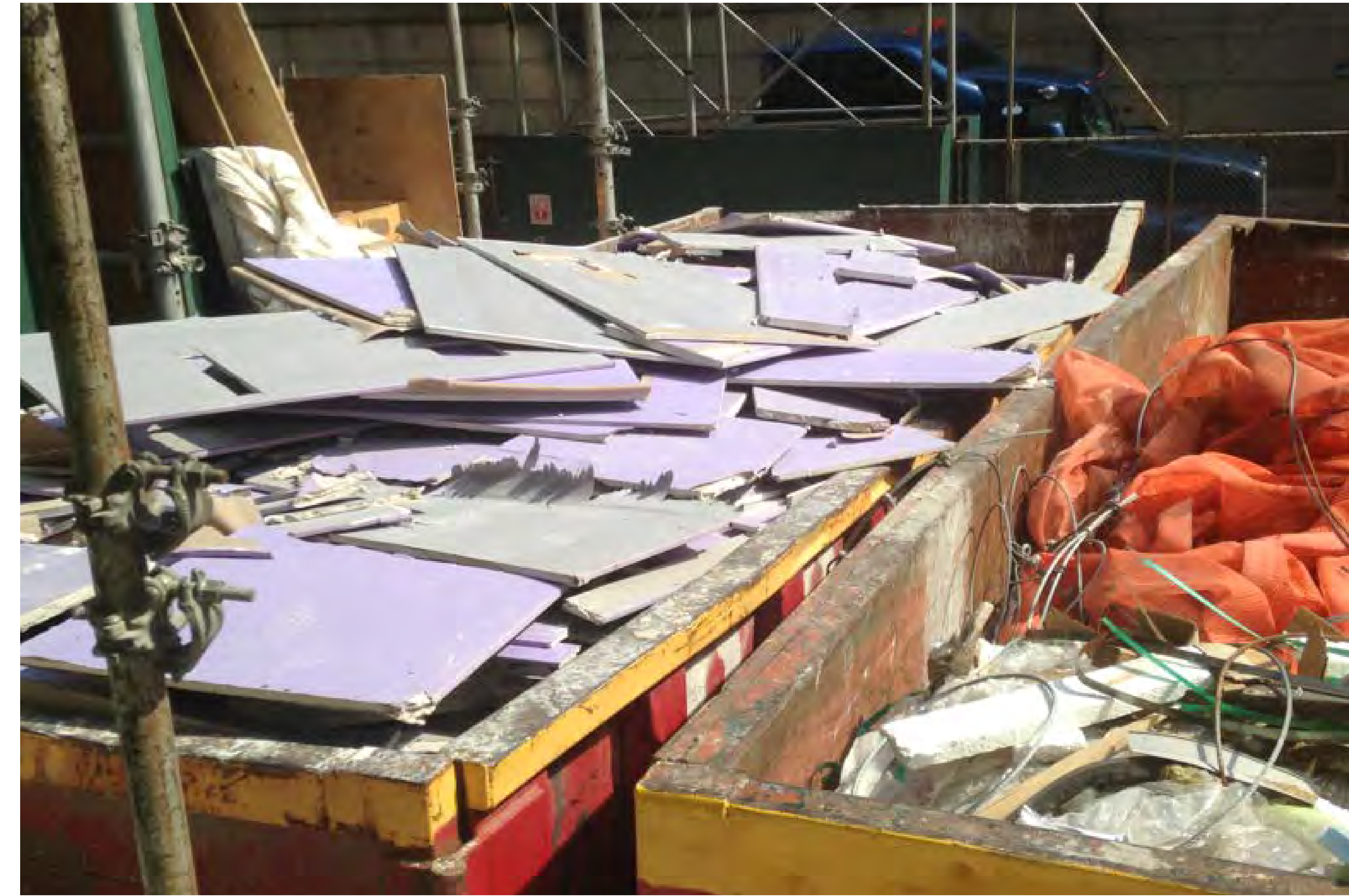
GWB scraps separated for recycling in 30 cu yd containers on a large construction site
