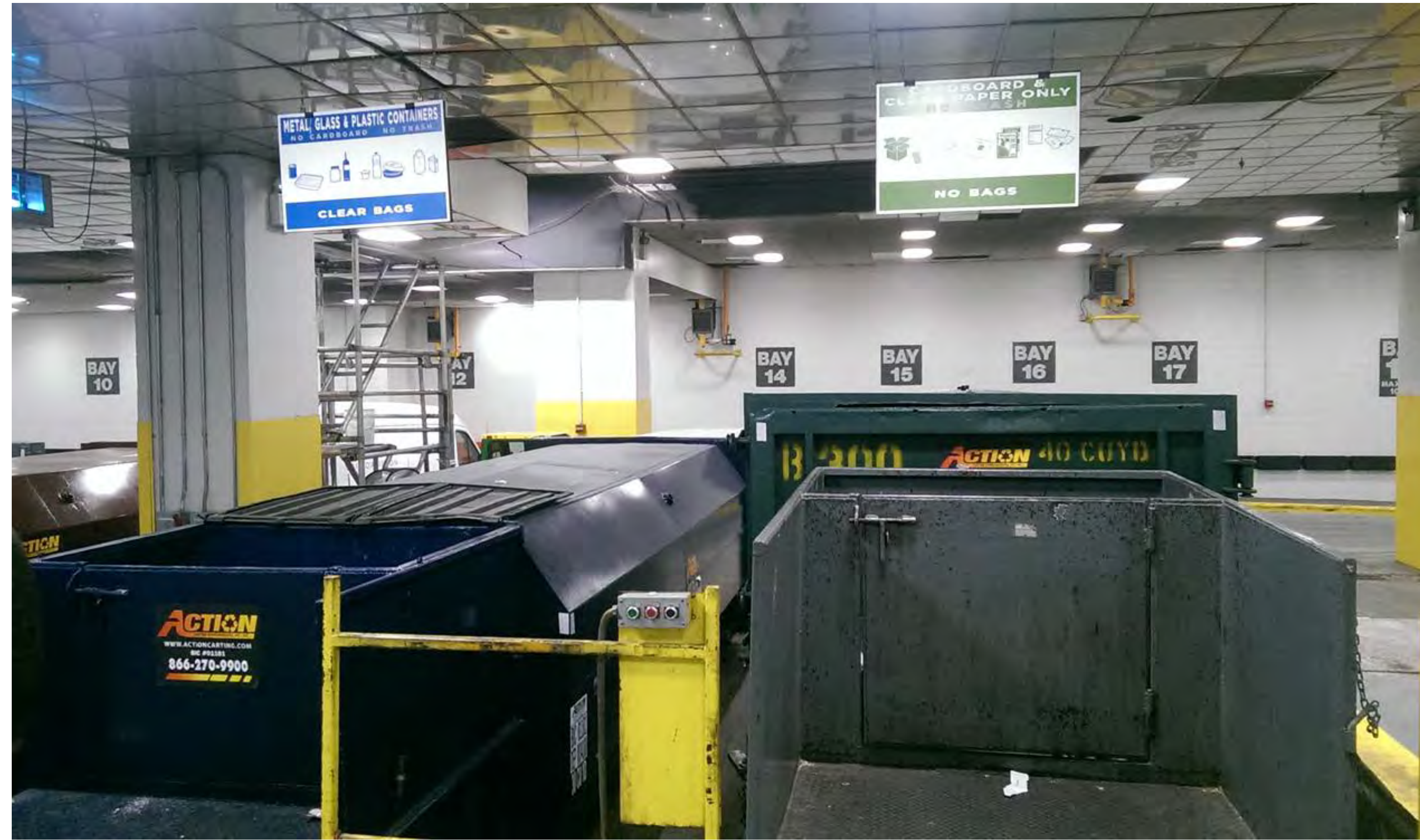
Loading dock with shared compactors for multiple waste streams
