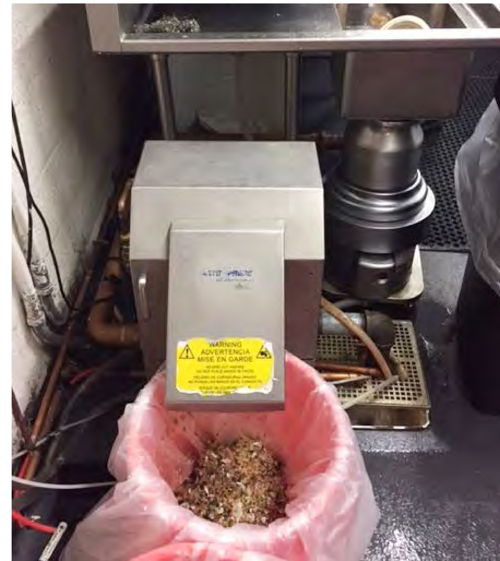
Clockwise from top left: Chemtracker collection bins for laboratory bottles; Central waste collection in courtyard; Pulper breaks down food waste for organic waste collection
