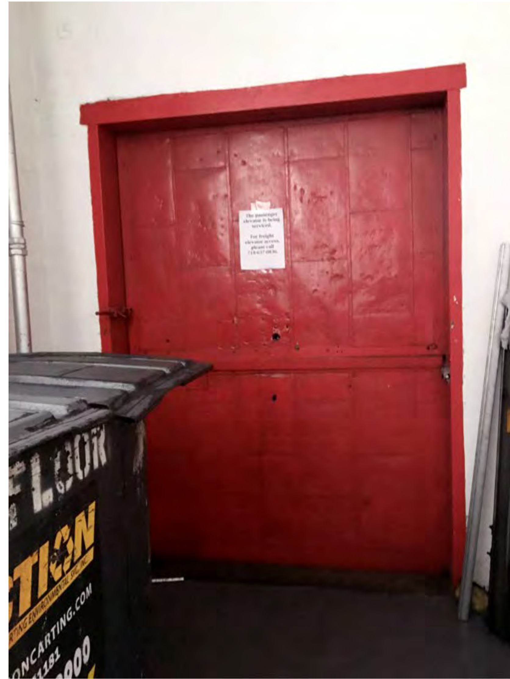
Clockwise from top left: Recycling being transferred from bin on dolly to tilt truck; Freight elevator takes tenant containers directly down to street; Service entrance to sidewalk freight elevator, door opens onto street
