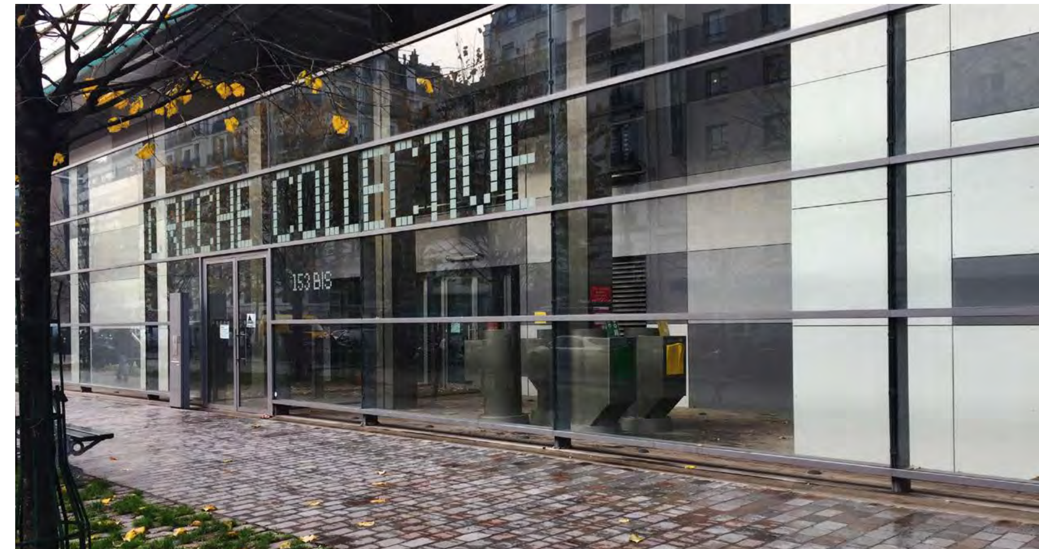
Top to bottom: Clichy-Batignolles eco-district; 153 bis rue Cardinet with pneumatic inlets for residents and daycare visible through facade
