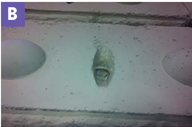
▲ Bunker block with rebar "hook" for stacking and moving.
