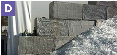
◀ Stair-stepped side wall of bunker, eliminating the need for half-blocks.
