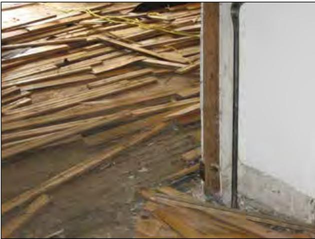
**Figure 5. Hardwood flooring boards being removed during deconstruction.**
