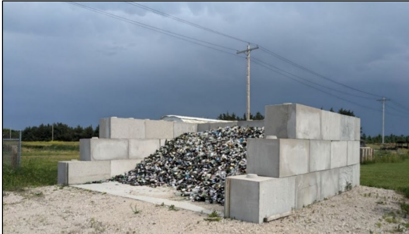
Figure 11: Village of Stuart glass recycling concrete bunker
